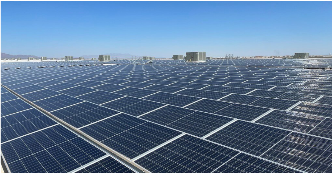
TJX’s distribution center in El Paso, TX features rooftop solar panels.
